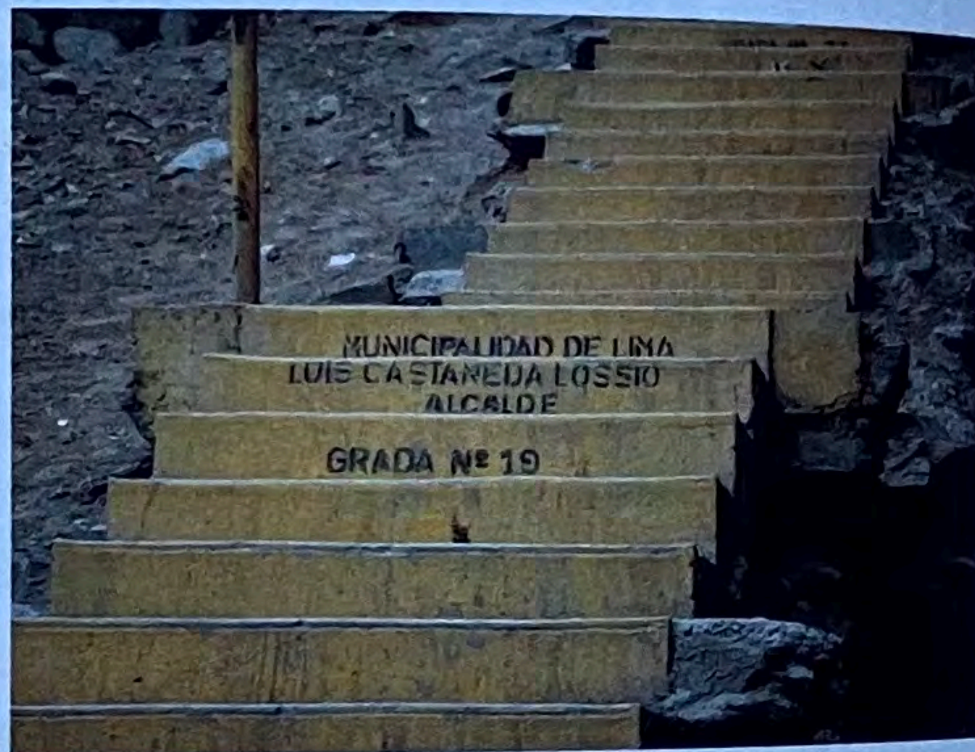
Fig. 3: Access and evacuation stairs in the Ate District.
